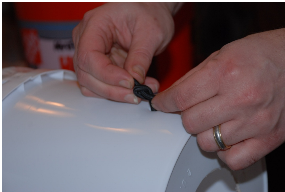
Figure 15 - Tie a knot in the bungee cords on the outside of the bucket. For the size bucket and bungee we used, there was about 1" of extra material after the knot. You may need to adjust the location of the knot to provide correct tension on the bungee. The cord should be slack with the plastic sheet pressed all the way in the bucket, but in tension when the sheet is pulled back.
