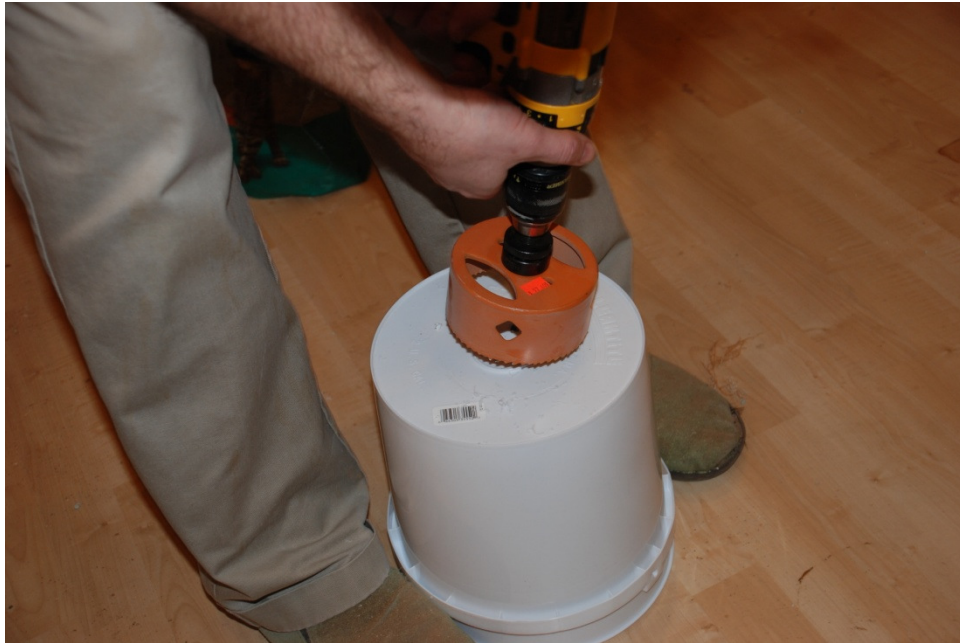
Figure 2 - Cut a hole about 6" diameter in the bottom of the bucket.... There's a hole in the bucket, dear liza.... If you don't have a 6" hole saw, just draw a circle with a compass or other round object and cut with a utility knife.
